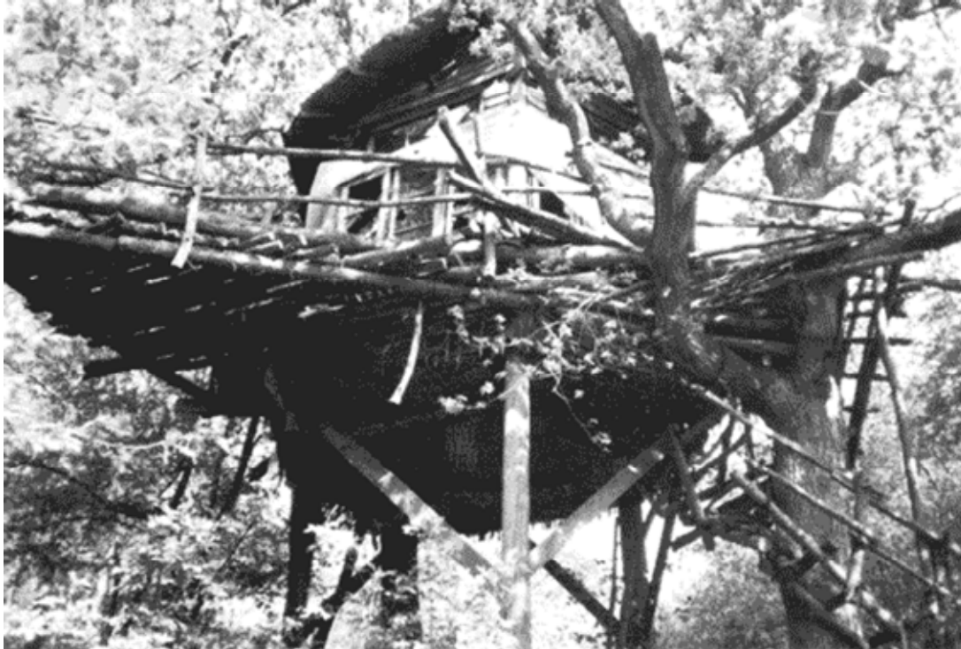
A view of the stairway and terrace from below, Chilham Woods
