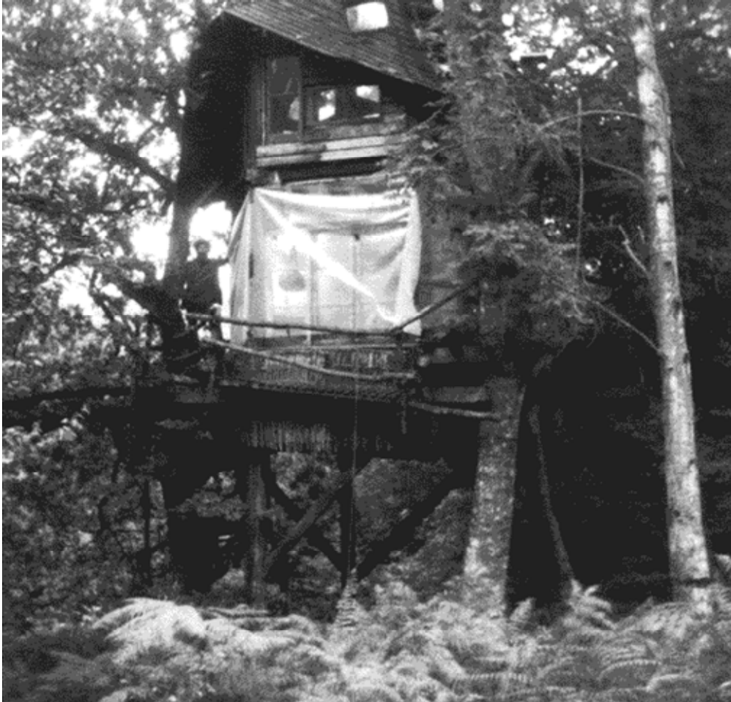
The lower floor of the treehouse in Chilham Woods is now protected by wraparound plastic
